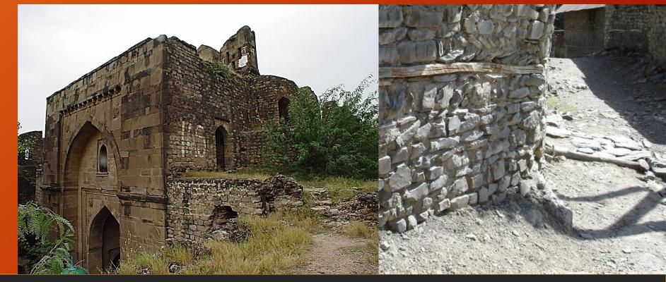
• The stone masonry in which either undressed or roughly dressed stones, are laid is called "Rubble Masonry".
