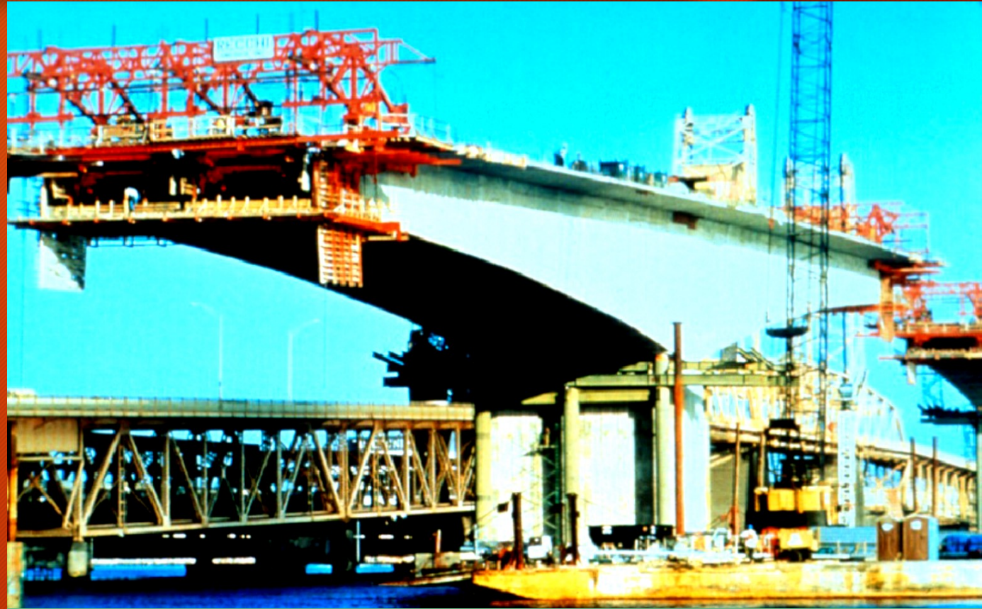
Cast-In-Place Segmental Construction using Form Travelers
