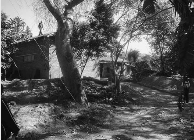
Figure 20.1 Disturbance associated with building activity in coastal forests. Building material introduced onto the site present a source of pollutants. A large opening was created in the forest canopy, which will remain indefinitely, and access roads with associated soil compaction will also affect tree root systems over the long term. These are examples of impacts of varying intensity and temporal scale.
